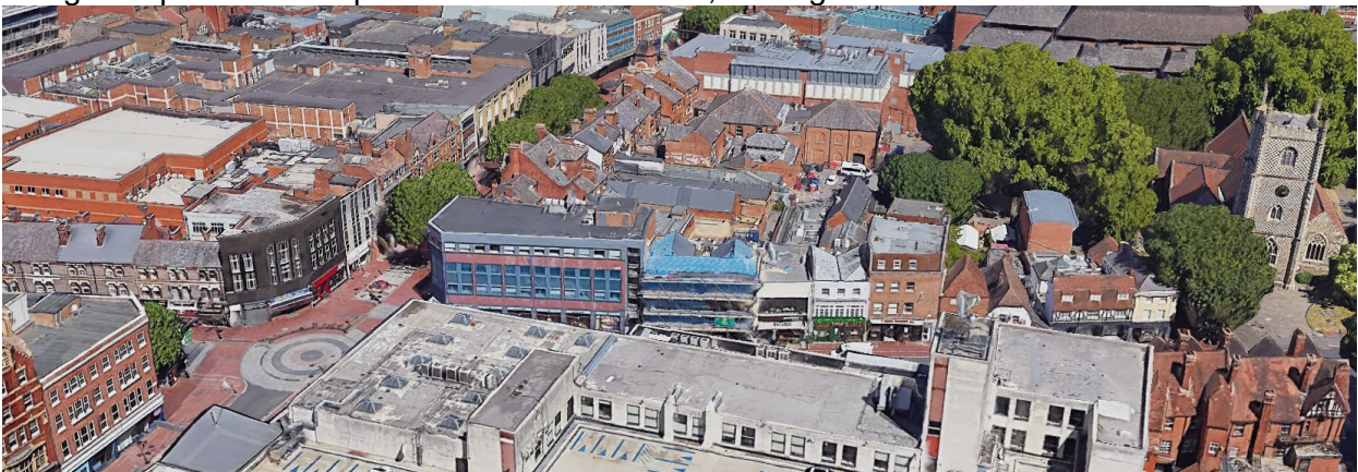
Google Maps aerial viewpoint from the west, showing the St Mary's Butts street elevation
